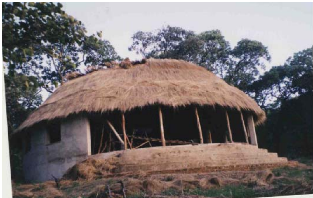
Figure 1 The meeting room at the Kasanka Research Centre nearing completion
